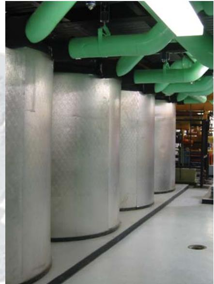
1155 Avenue of the Americas, a 41-story building in New York City, is cooled by twenty-eight IceBank® Storage tanks. The tanks have a capacity of 3200 ton-hours.
